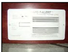
Figure 4-22. Carbon Monoxide/LP Gas Detector
