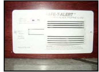
**Figure 3-6. CO/LP Gas Detector**
